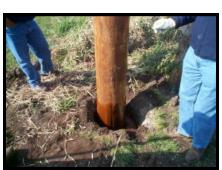
work in all soil conditions, including wet areas. Poly-Set bonds tightly to all pole types (i.e. wood, steel, composite, and concrete). It fills in all voids in the hole created by the excavation process. Poly-Set is supplied in various kit sizes to accommodate the installation or repair application from straightening poles to setting brand new poles.
